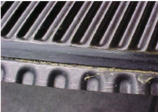
Old glue has not been removed from the gasket groove prior to regasketing.
