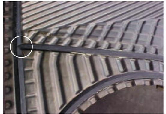
The use of excess glue contributed to diagonal gasket movement shown here within the ringed area.
