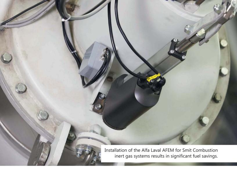
The Alfa Laval Automatic Fuel Efficiency Module (AFEM) is a new modification for reducing the fuel consumption of Alfa Laval Smit Combustion inert gas systems by ensuring the inert gas that keeps cargo safe during offloading is only generated in the exact amounts required. In a two-year pilot project, the AFEM allowed Italian shipping company Navigazione Montanari S.p.A. to achieve average fuel savings of 30 per cent.
